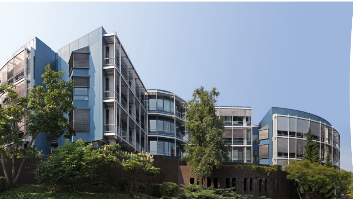
Thieme Headquarter in Stuttgart, Germany
